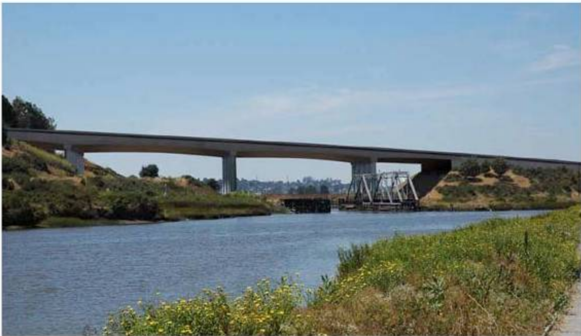
Figure 3.1-40 Simulation of Proposed Petaluma River Bridge Design (Pre-cast Tee Girder Option)
