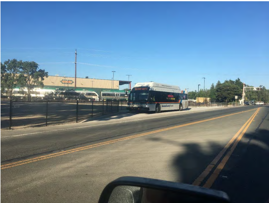
Joint Project with Sonoma County - New bus pull-out and sidewalk at the Airport Station parking lot
