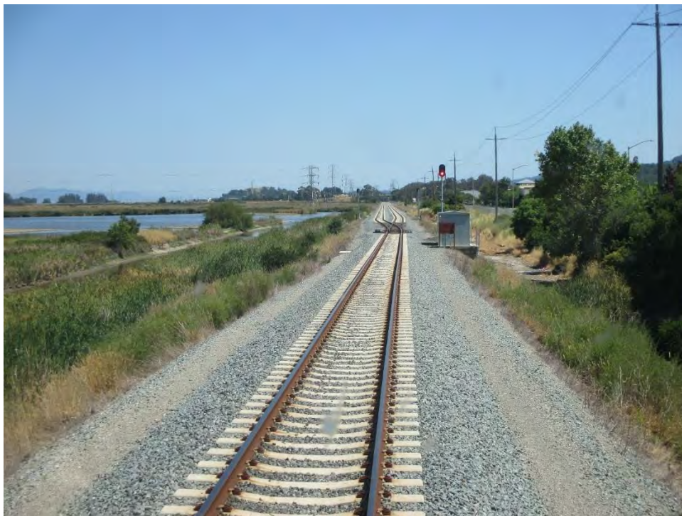
Approaching red signal at Control Point Ignacio North during Operational Testing, Novato
