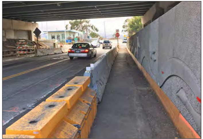
Widening undercrossing of Highway 101 to provide additional traffic lanes.
