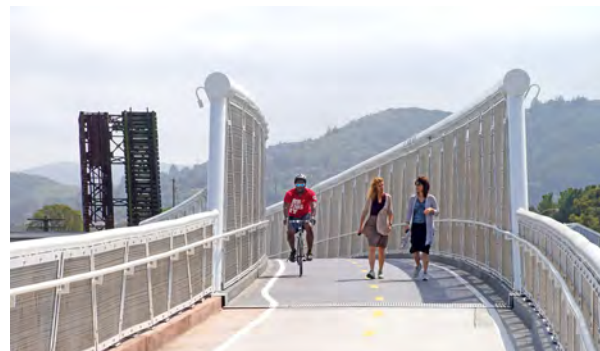
The recently opened Central Marin Ferry Connector in Larkspur
