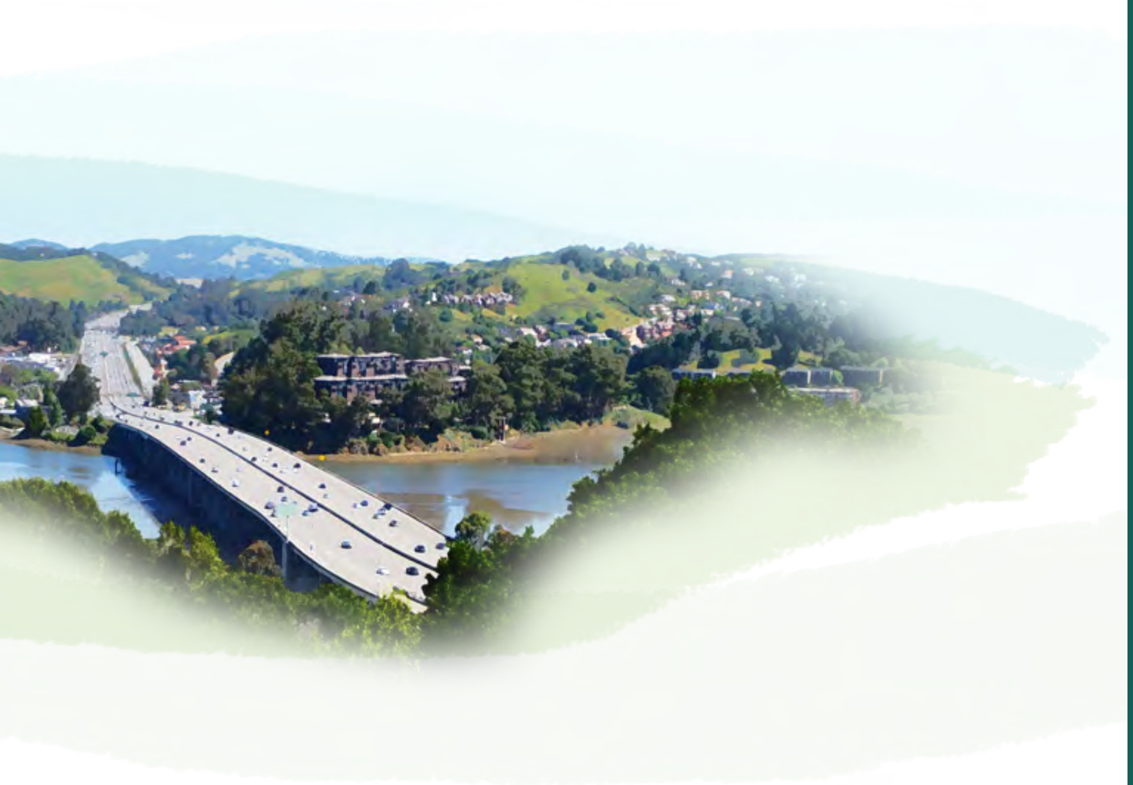
Highway 101 over Richardson Bay in Southern Marin
