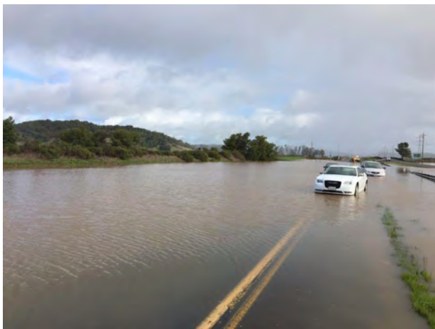
Highway 37 flooded in Marin during winter 2017
