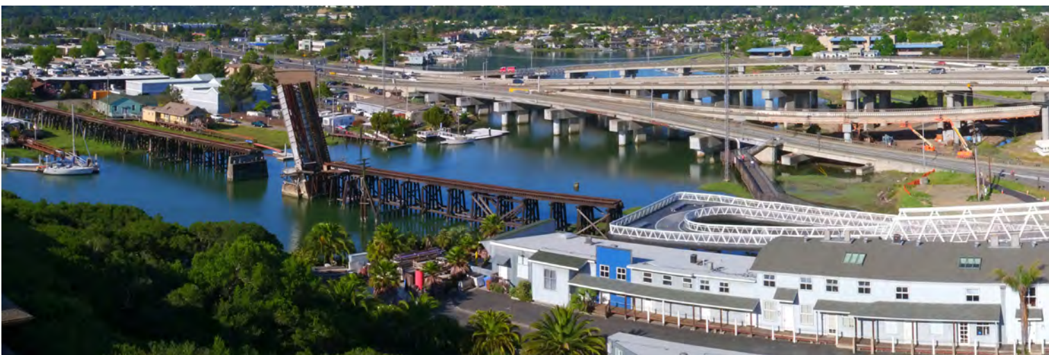
Aerial view of the Central Marin Ferry Connector
