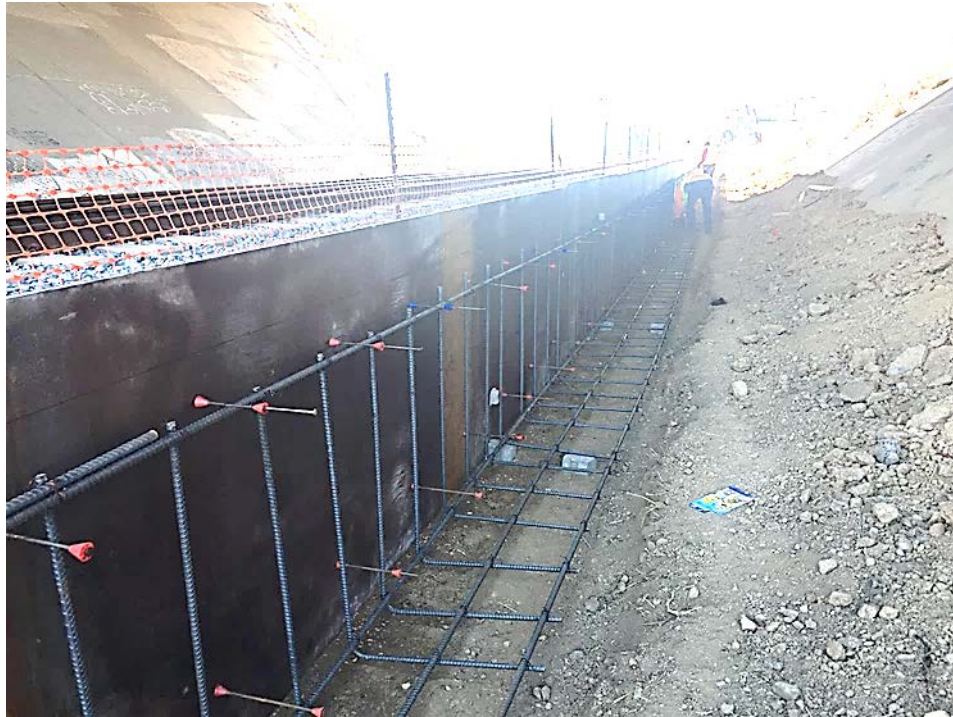
Crews construct the retaining wall north of Rush Creek Place (Novato) that will support the pathway.
