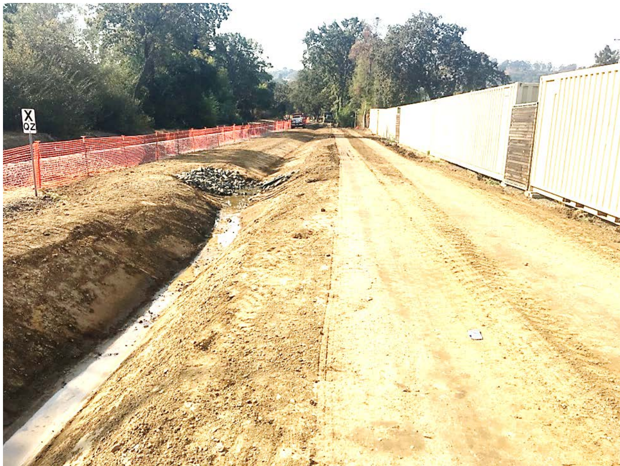
The pathway north of North San Pedro (San Rafael) before crews finished paving.
