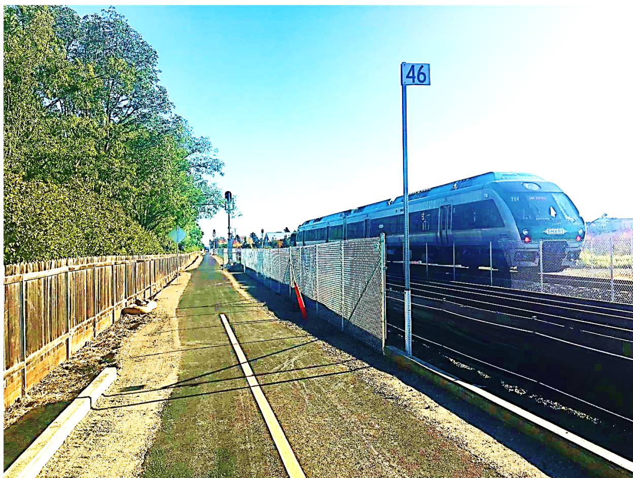
Completed pathway south of the Cotati Station.
