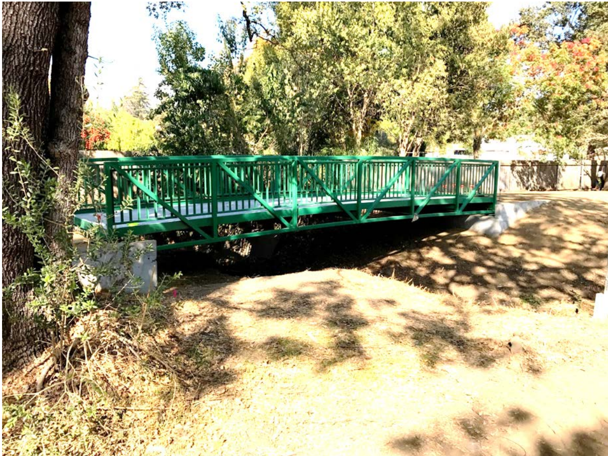
Pedestrian pathway bridge south of the Civic Center Station has been installed.
