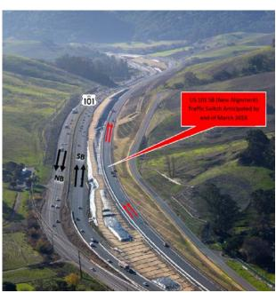
Construction crews are preparing for a traffic shift of southbound traffic on the Marin-Sonoma Narrows project at the Marin-Sonoma county line. Motorists can see construction progressing on the future roadway alignment and the new bridge over San Antonio Creek. In March, southbound traffic will be shifted to the west and onto the new bridge that was completed in December. A video of the recent concrete pour for the new bridge deck is available on the www.tam.ca.gov website.
