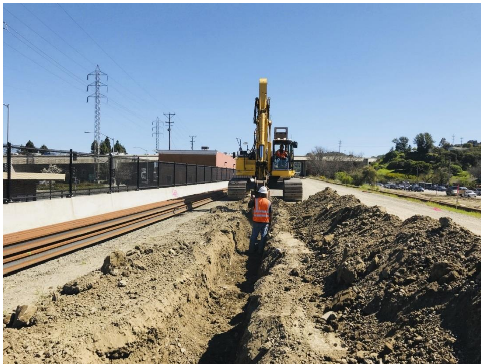
Ductbak Installation between Auburn Street and Andersen Drive
