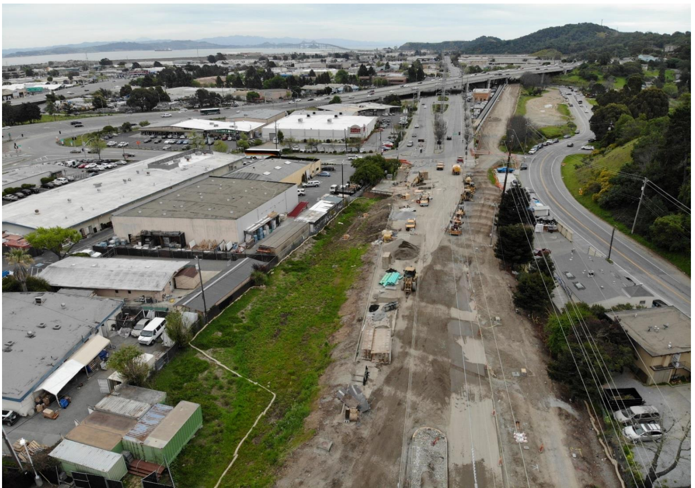
Aerial view of Andersen Drive Construction
