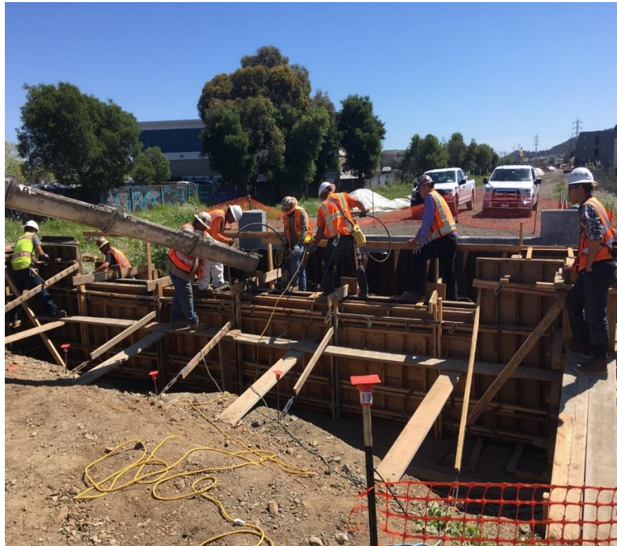
Concrete placement for the north bridge abutment at the Unnmaed Channel
