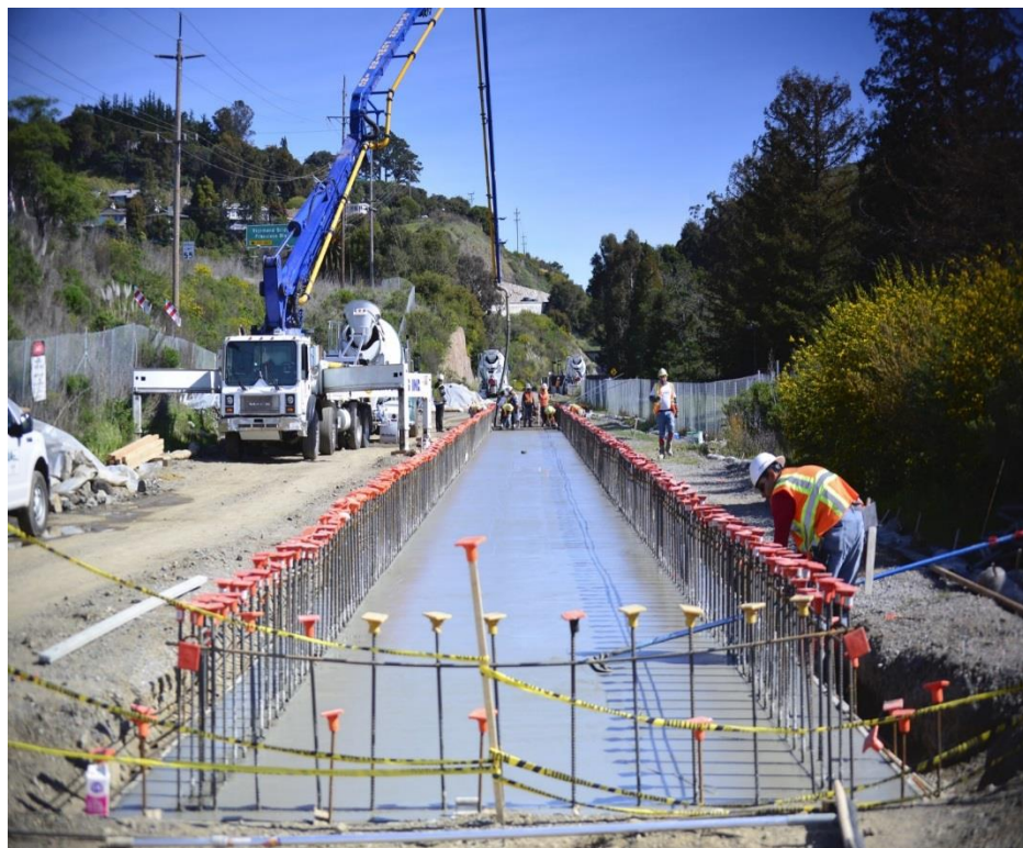
Larkspur station Platform construction
