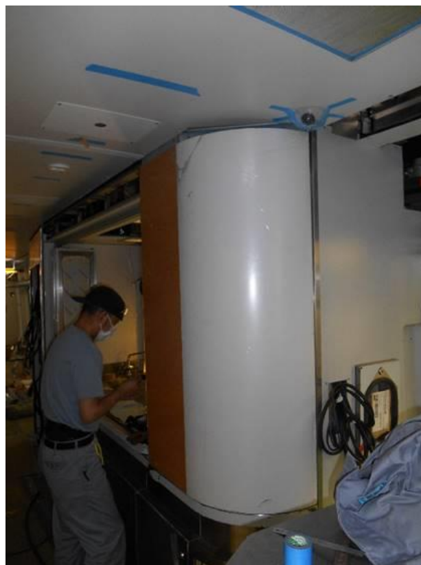
Car 117: Service Bar nearing completion
