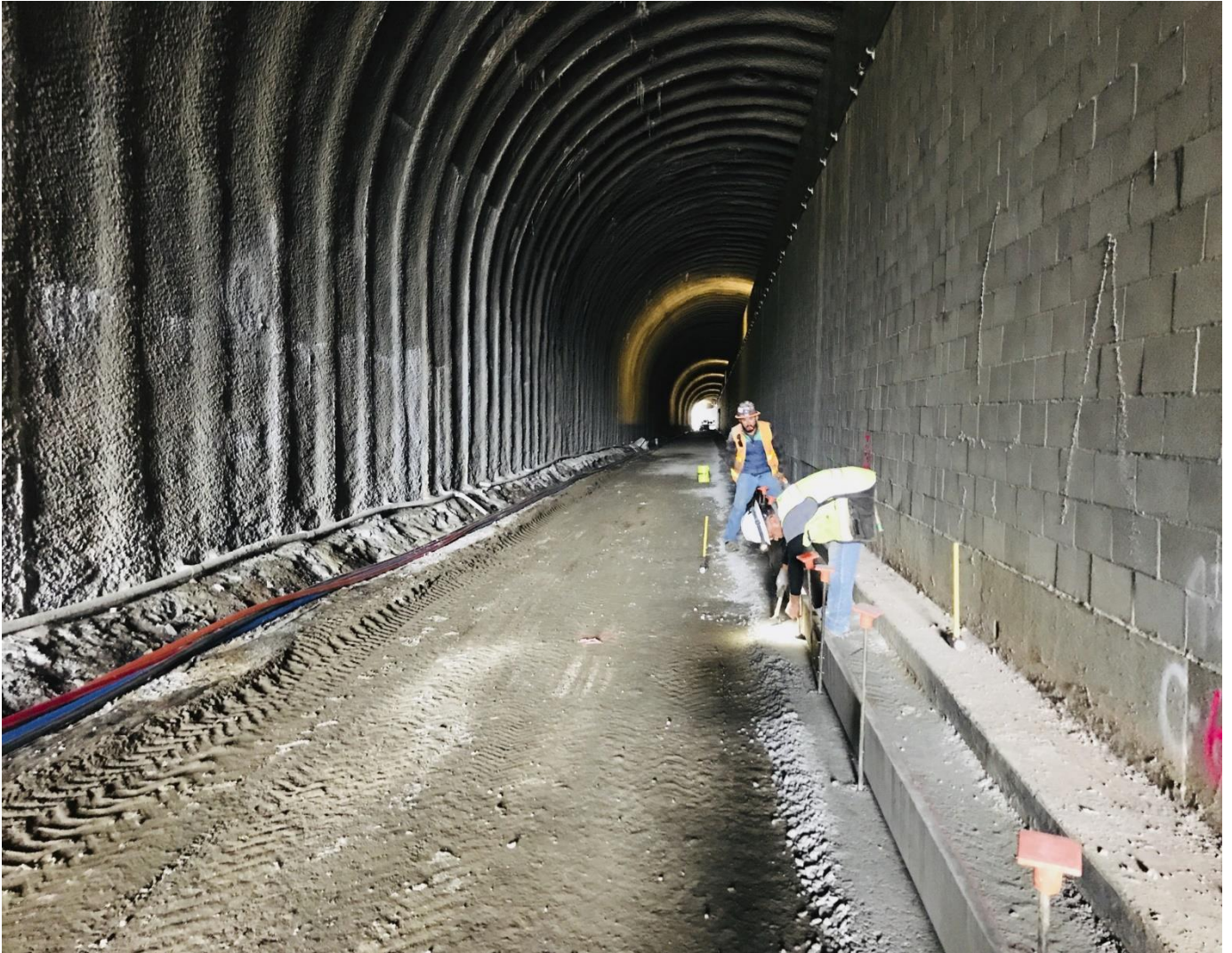
Cal Park Tunnel grading work
