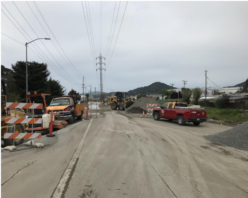
Andersen Drive construction
