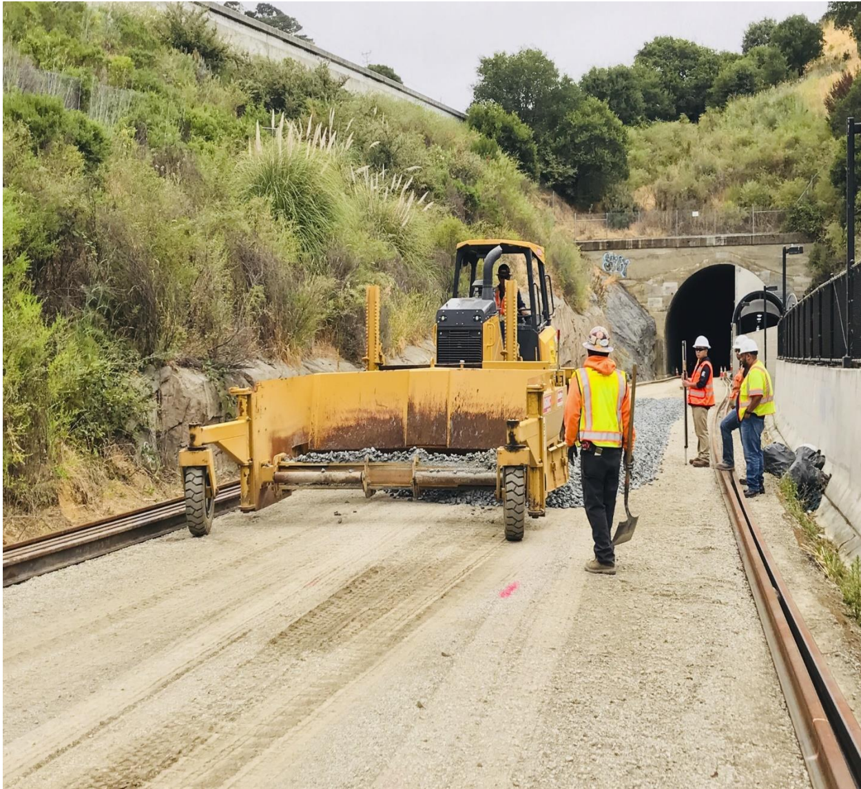
South Cal Park Tunnel to Station placing the gravel ballast for the track
