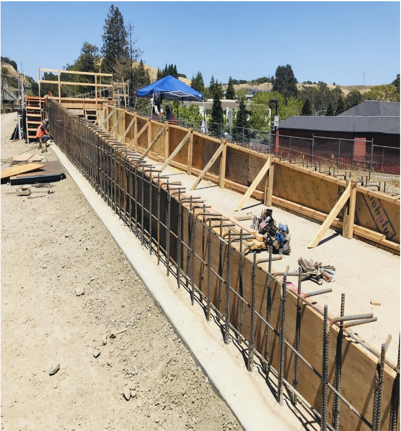
Larkspur Station Platform Ramp – concrete formwork
