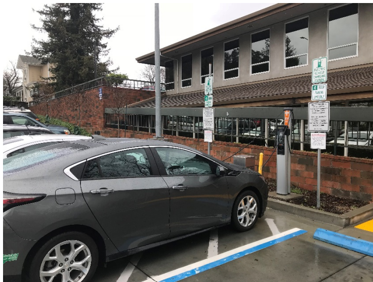
Public Charging Station Located in downtown San Rafael
