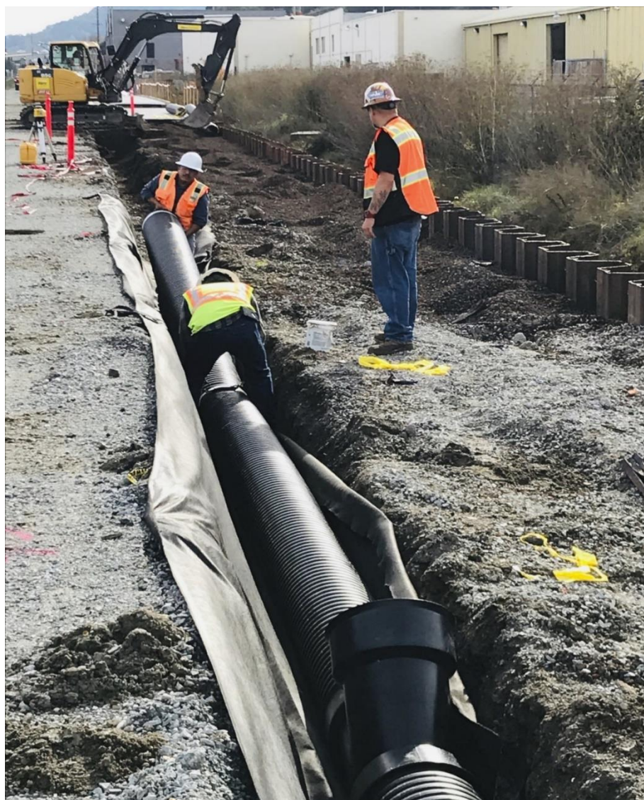
Installing 12" underdrain pipe between the track and the multi-use pathway.
