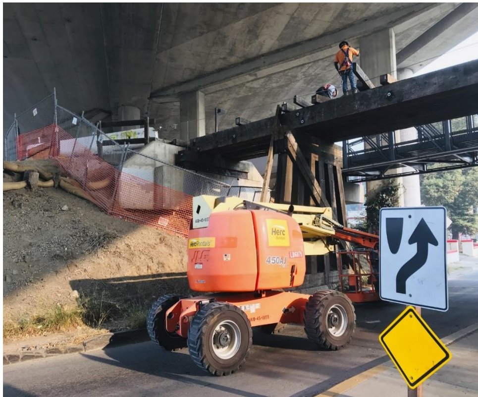
Installing deck timbers at the Auburn Street Trestle.
