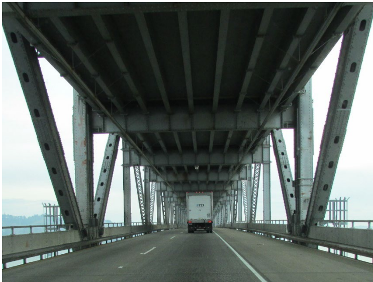
Lower Deck Shoulder Lane operating since April 2018
