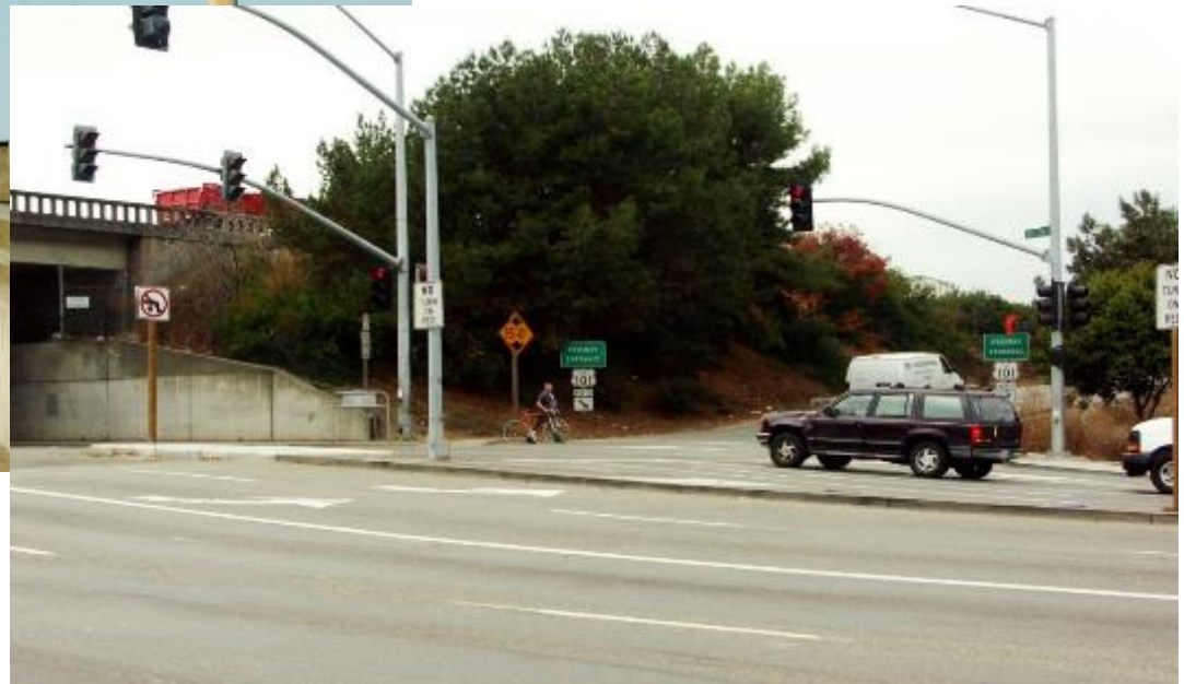
Widen Bellam Blvd Off-Ramp
