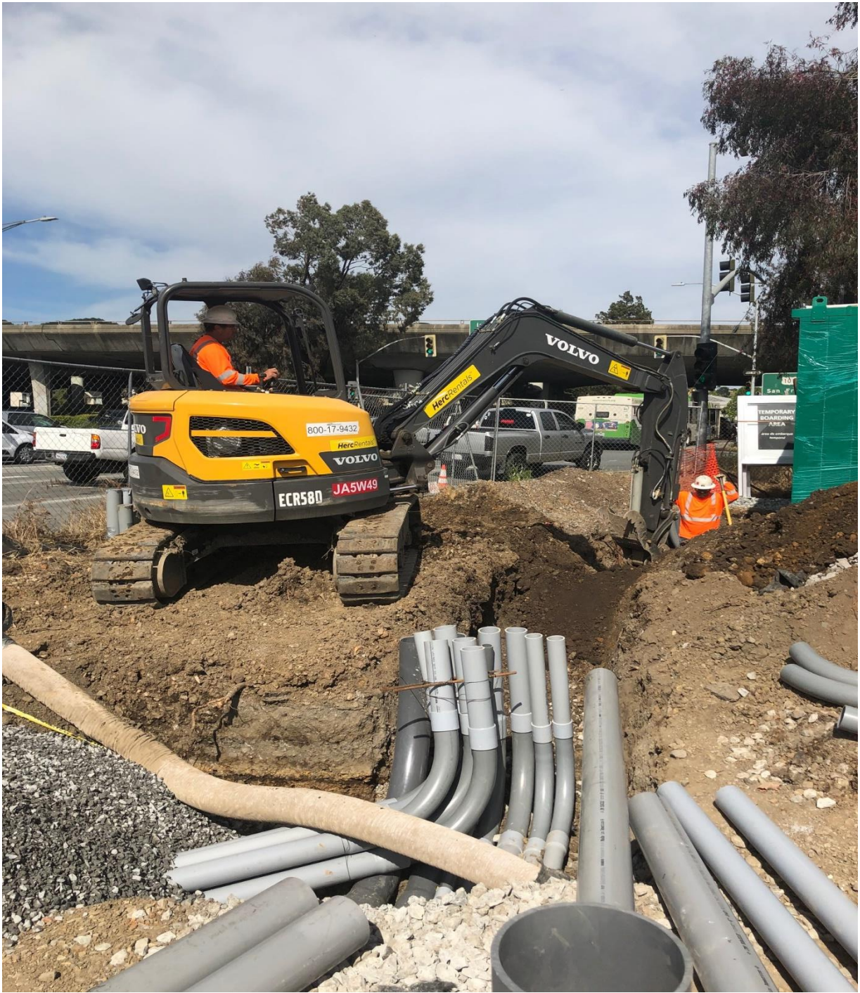
Signal conduit installation at 2 nd Street
