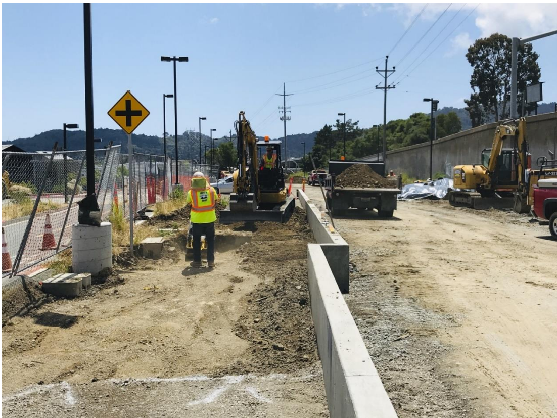
Larkspur Station- Ramp Construction
