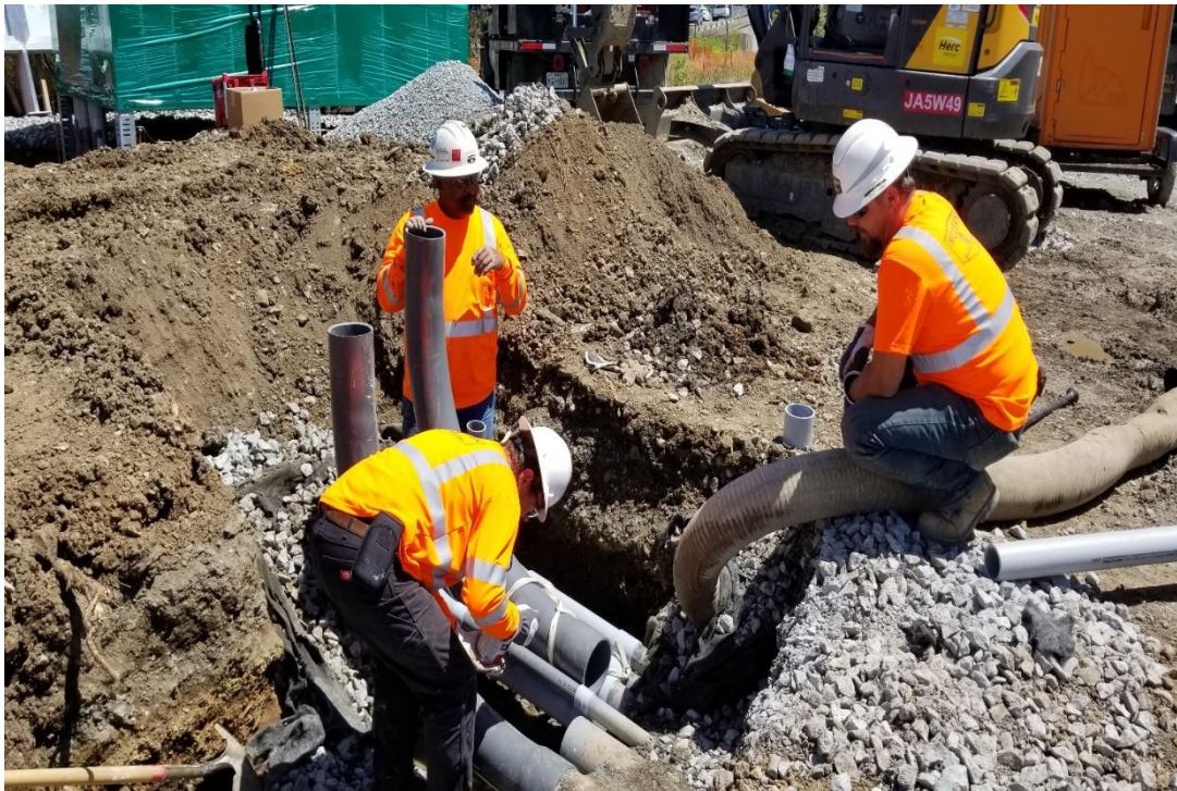
Conduit installation at the 2 nd Street
