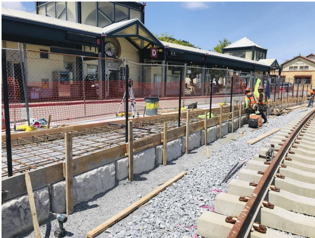
Bettini Transit Center – Track and concrete wall construction
