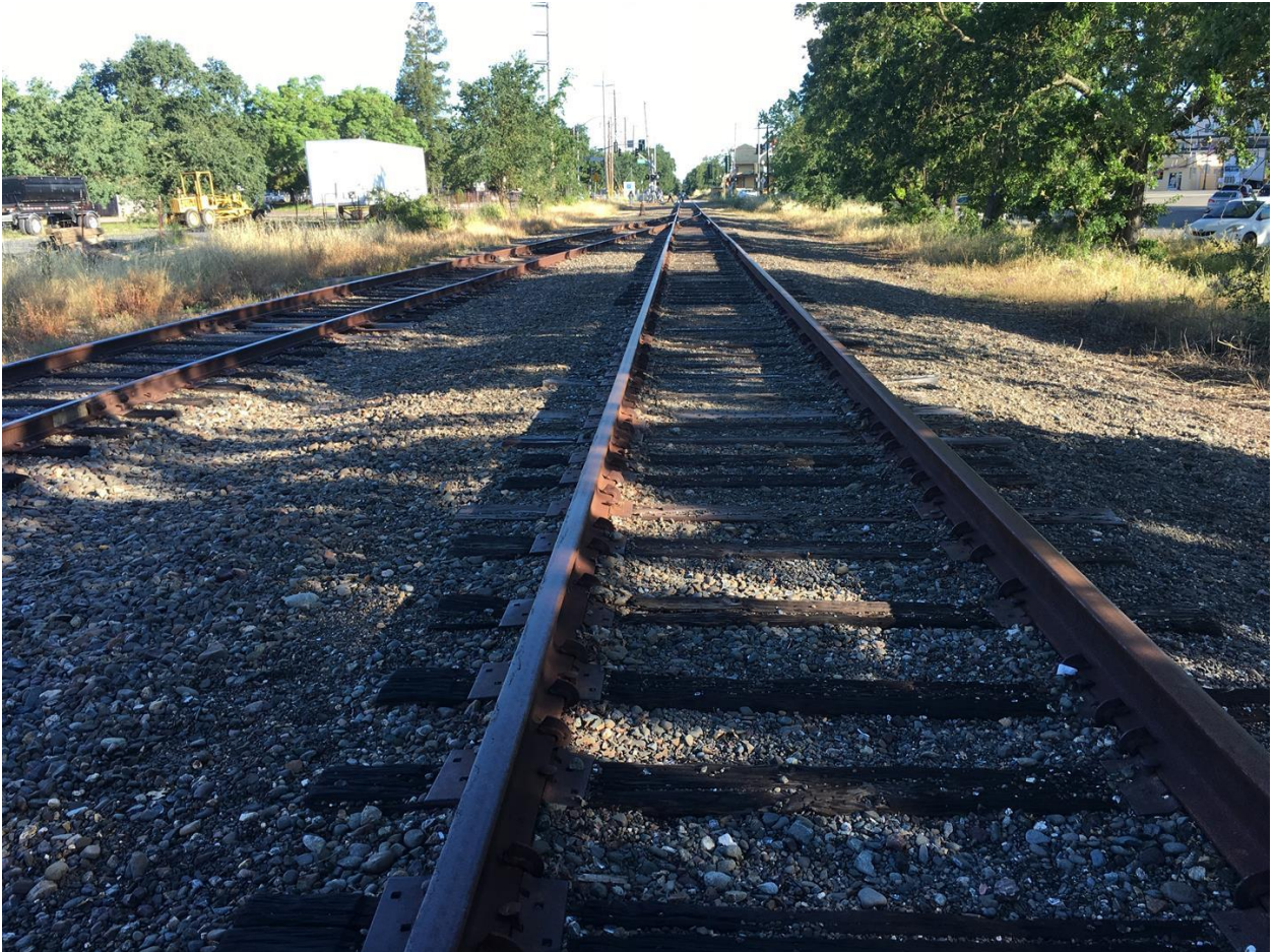
Windsor Extension- Looking north at Windsor River Road Crossing
