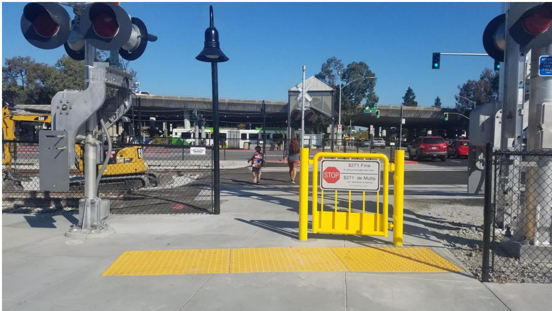
Bettini Transit Center – Pedestrian Safety channelization along 2 nd Street
