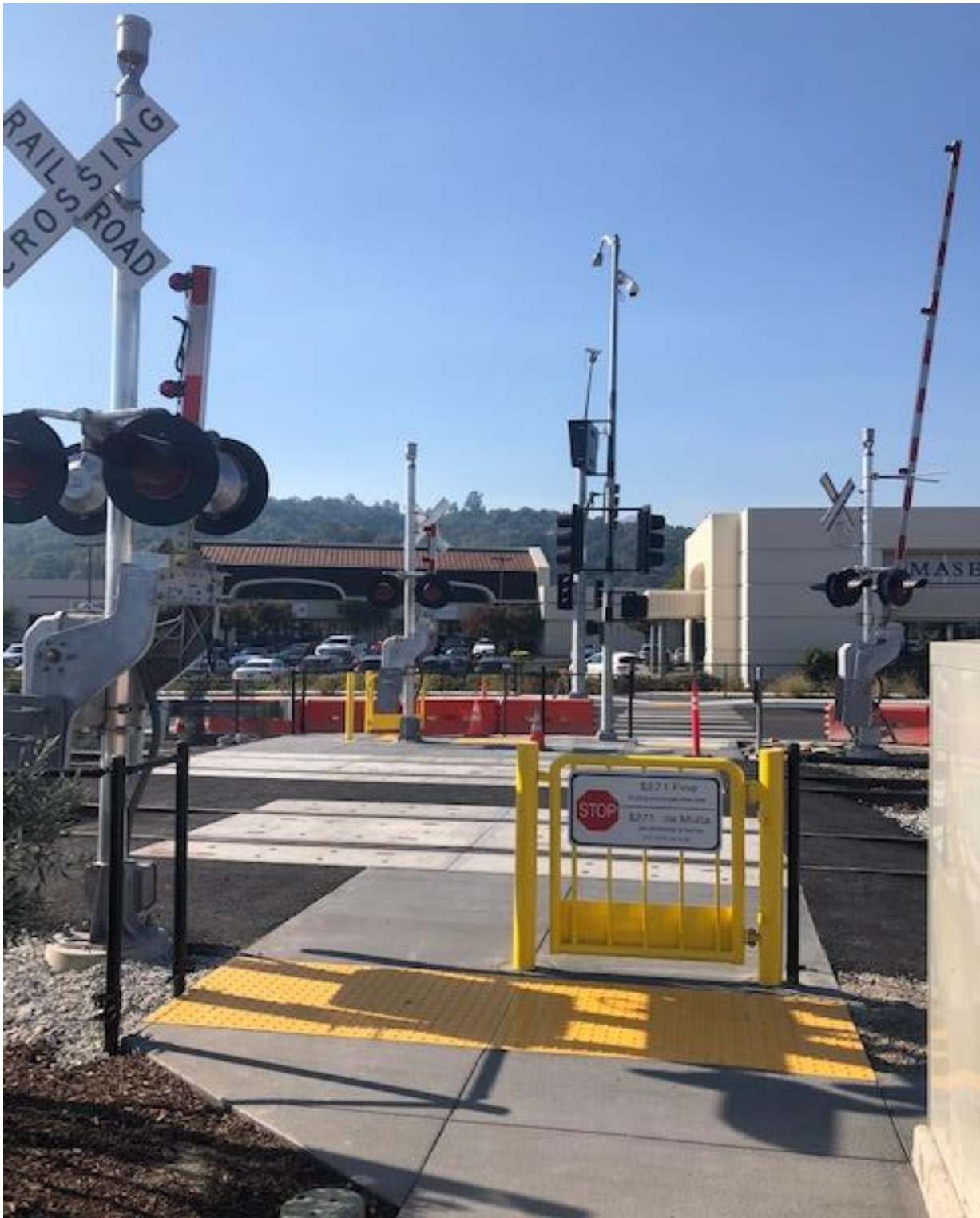
Francisco Boulevard Pedestrian Safety Enhancements Installation
