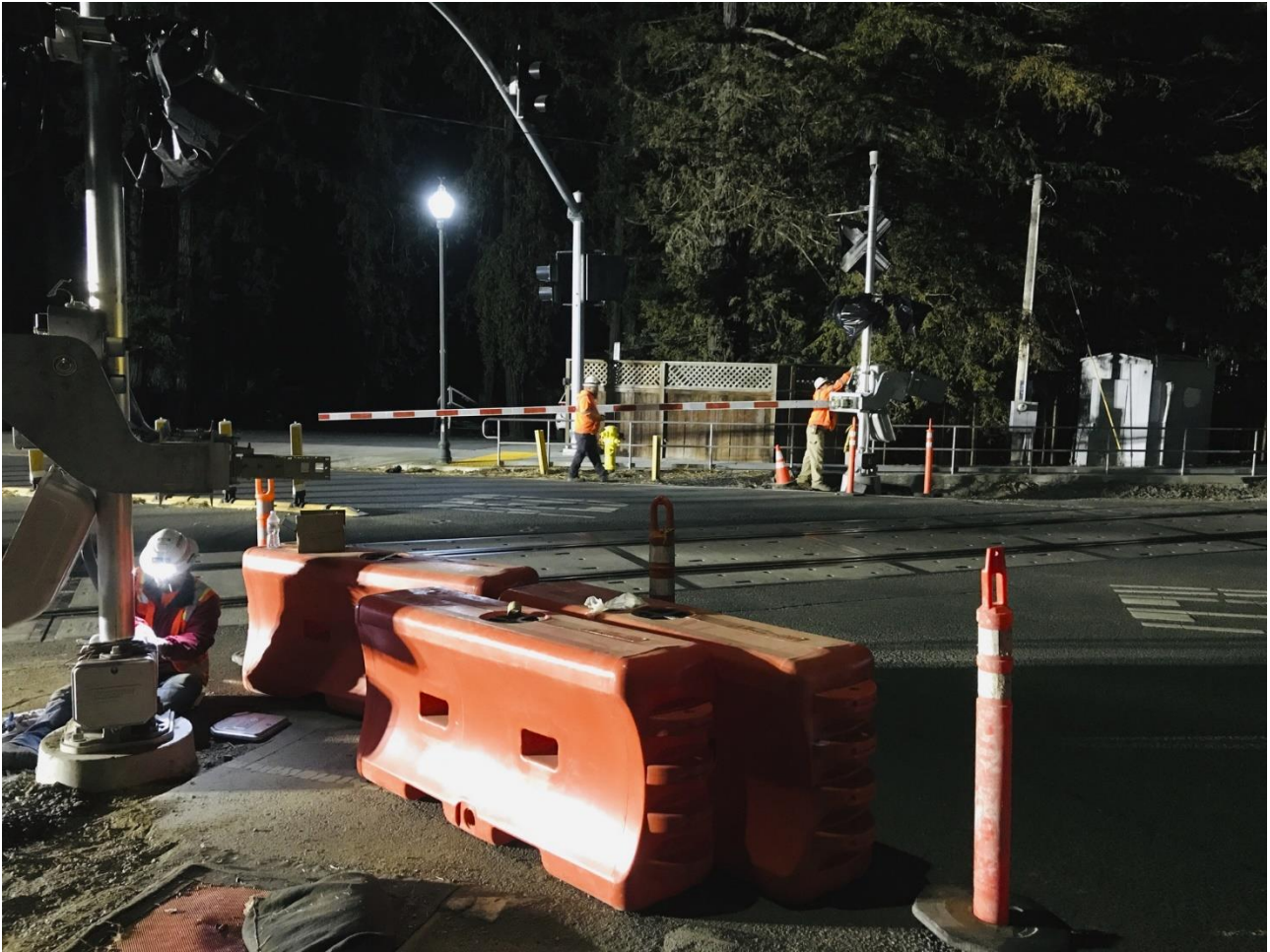
Main Street in Penngrove – installation of additional enhancement warning system gates
