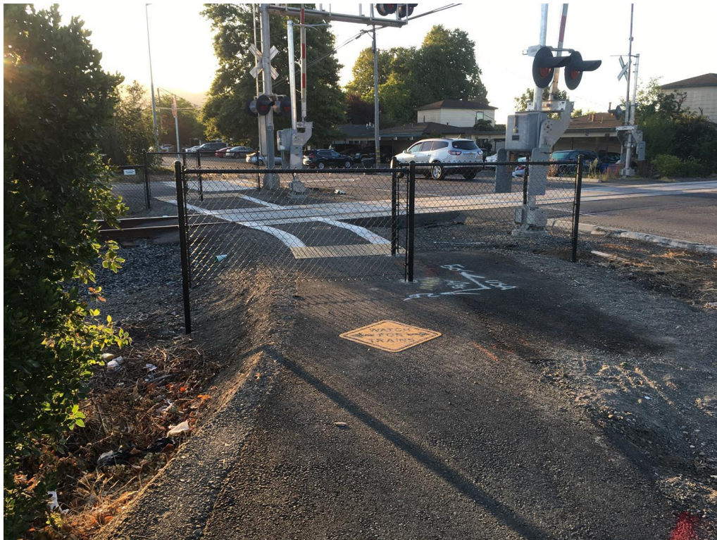
Bellevue Ave, Santa Rosa - Pedestrian Channelizing Fence
