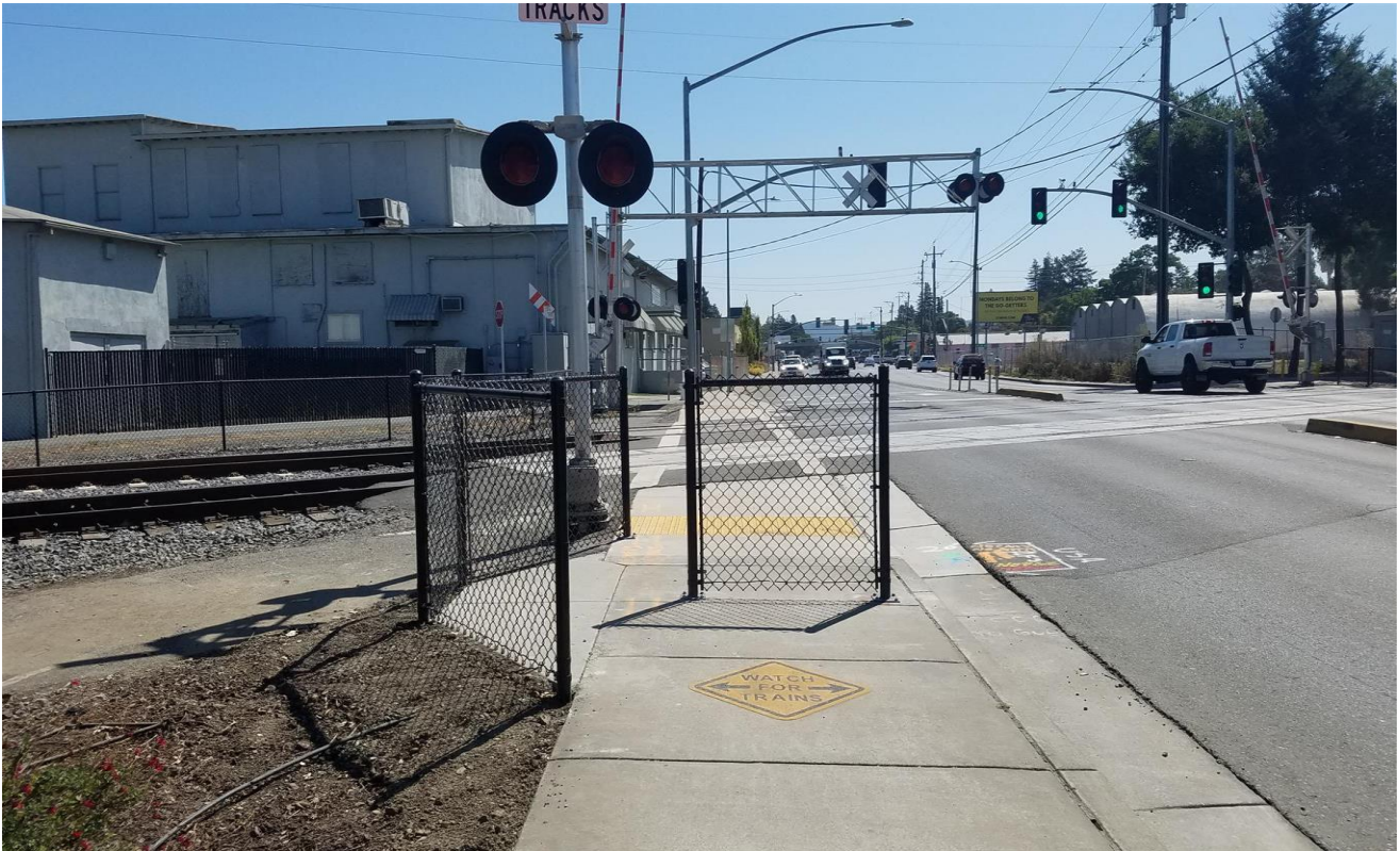
College Ave, Santa Rosa- Pedestrian Channelizing Fence
