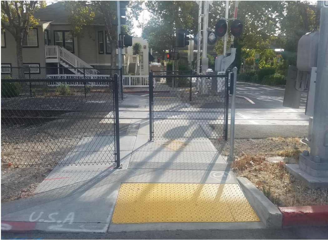
5 th Street, San Rafael - Pedestrian Channelizing Fence
