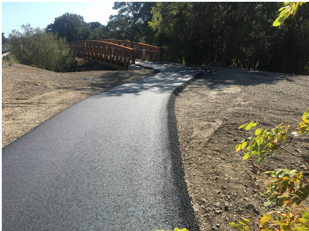
Paving North of the Petaluma River
