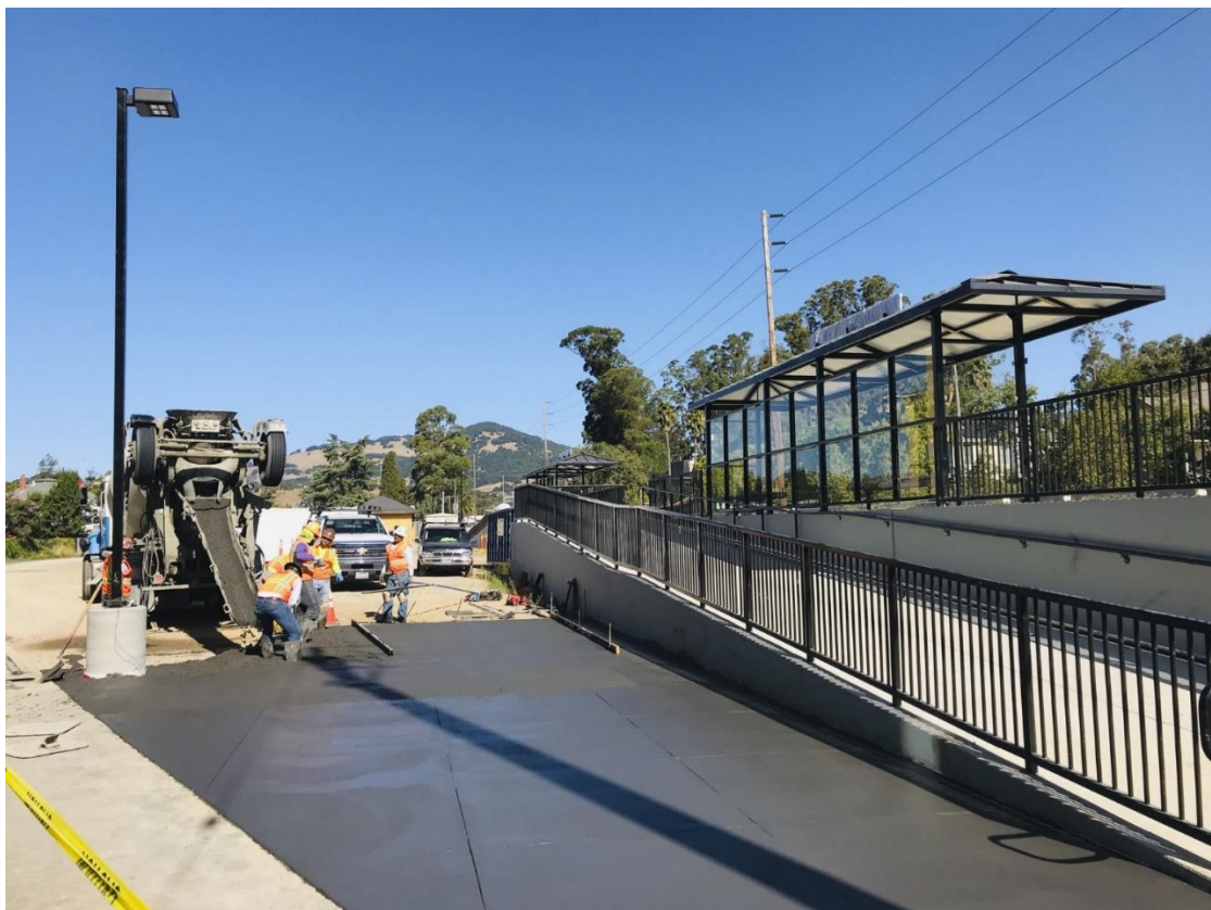
Novato Downtown Platform – Construction of Bicycle
