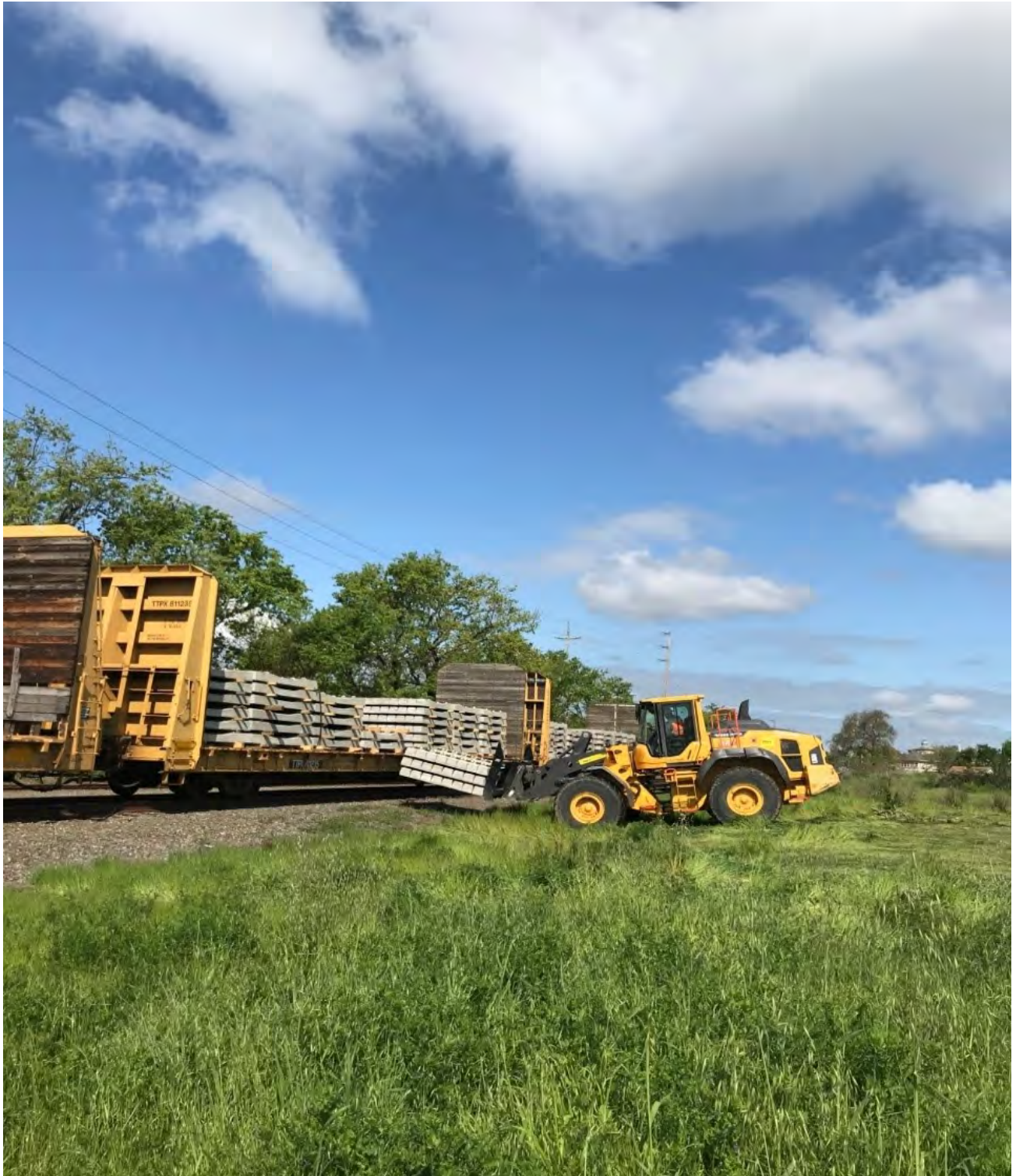
Concrete Tie Delivery
