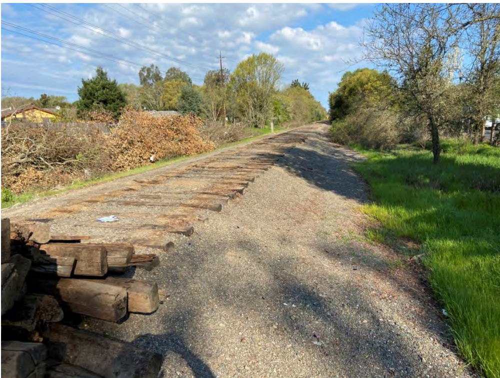
Track Demolition North of the Windsor Station
