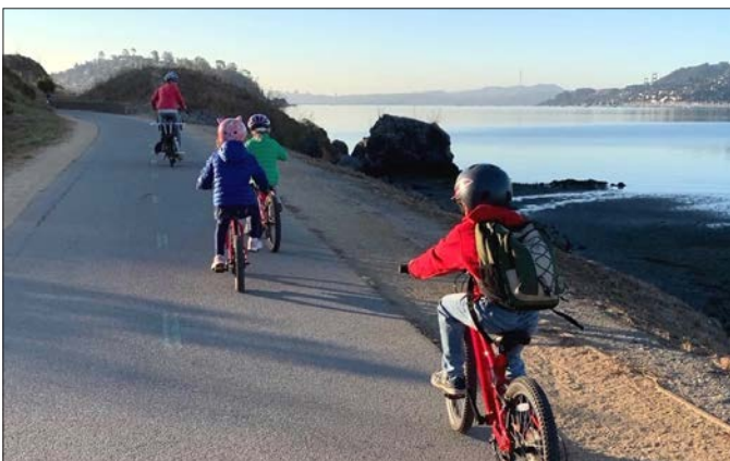
Multi-use pathways are shared between pedestrians and bicyclists and allow them to travel separated from vehicular traffic. Paths are typically at least ten feet wide to provide bi-directional travel.
