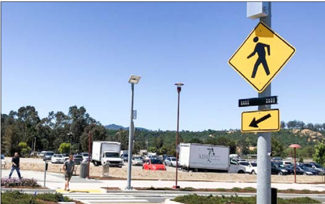
Rectangular rapid flashing beacons are pedestrian-activated beacons that supplement warning signs. By alerting motorists of pedestrians waiting to cross the street, they have been proven to increase driver yield compliance.
