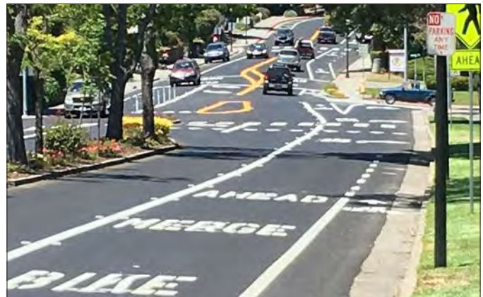
Bicycle lanes designate an exclusive space for cyclists through the use of pavement markings and signage. Bike lanes visually remind motorists of bicyclists' right to the street.
