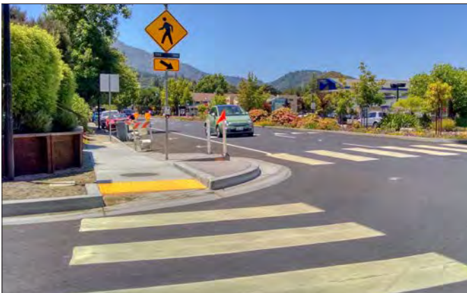
High-visibility crosswalk striping provides heightened visibility over standard crosswalk markings.
