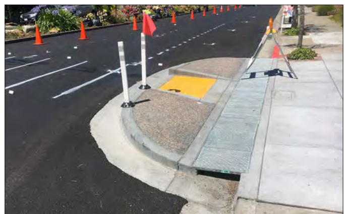
Curb extensions , sometimes called bulb-outs, make pedestrians more visible to motorists while providing additional room to wait before crossing the street. The extensions also reduce crosswalk lengths and slow turning vehicles.
