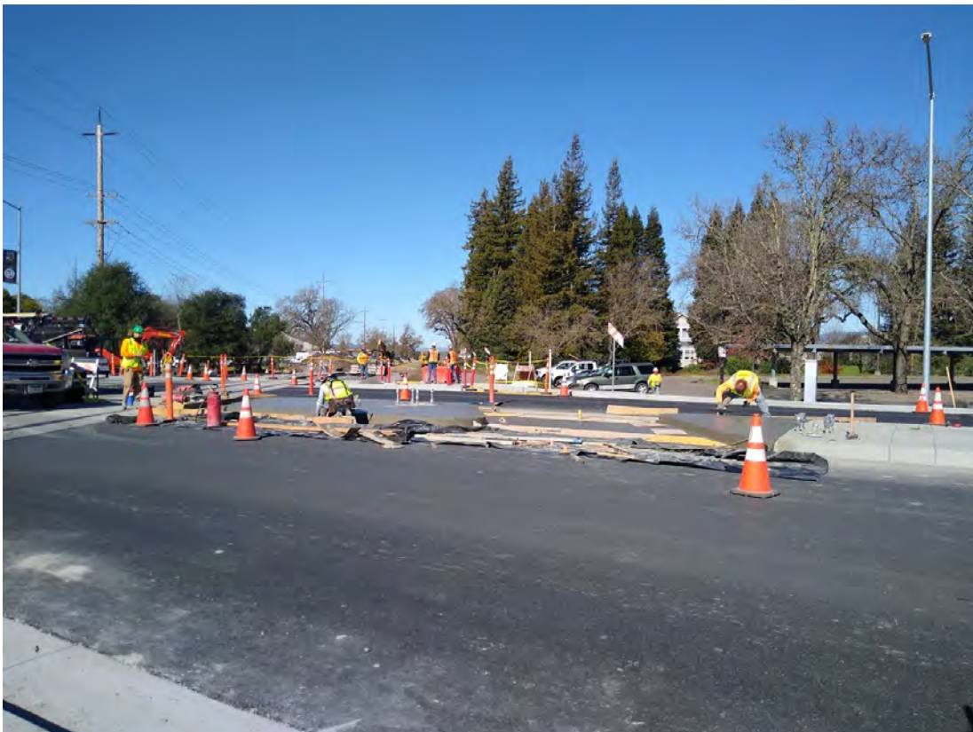
Airport Boulevard - Constructing Roadway Medians
