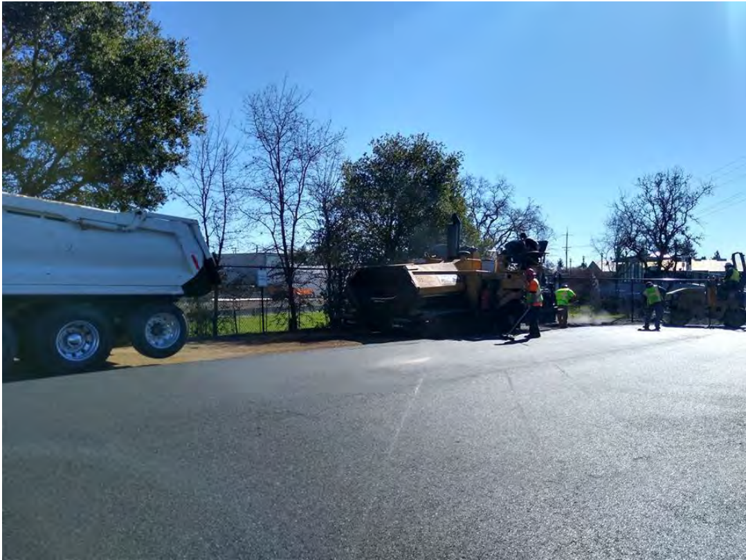
SMART Airport Station Parking Lot Paving
