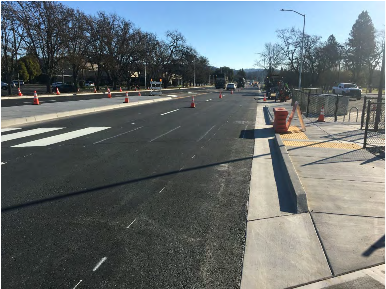
Airport Boulevard Crossing – Street Striping Being Installed
