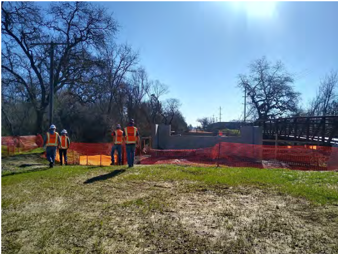
Site Walk Inspection with SMART Staff and the Contractor
