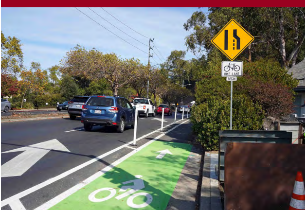
Major Roads projects continue to make major progress
