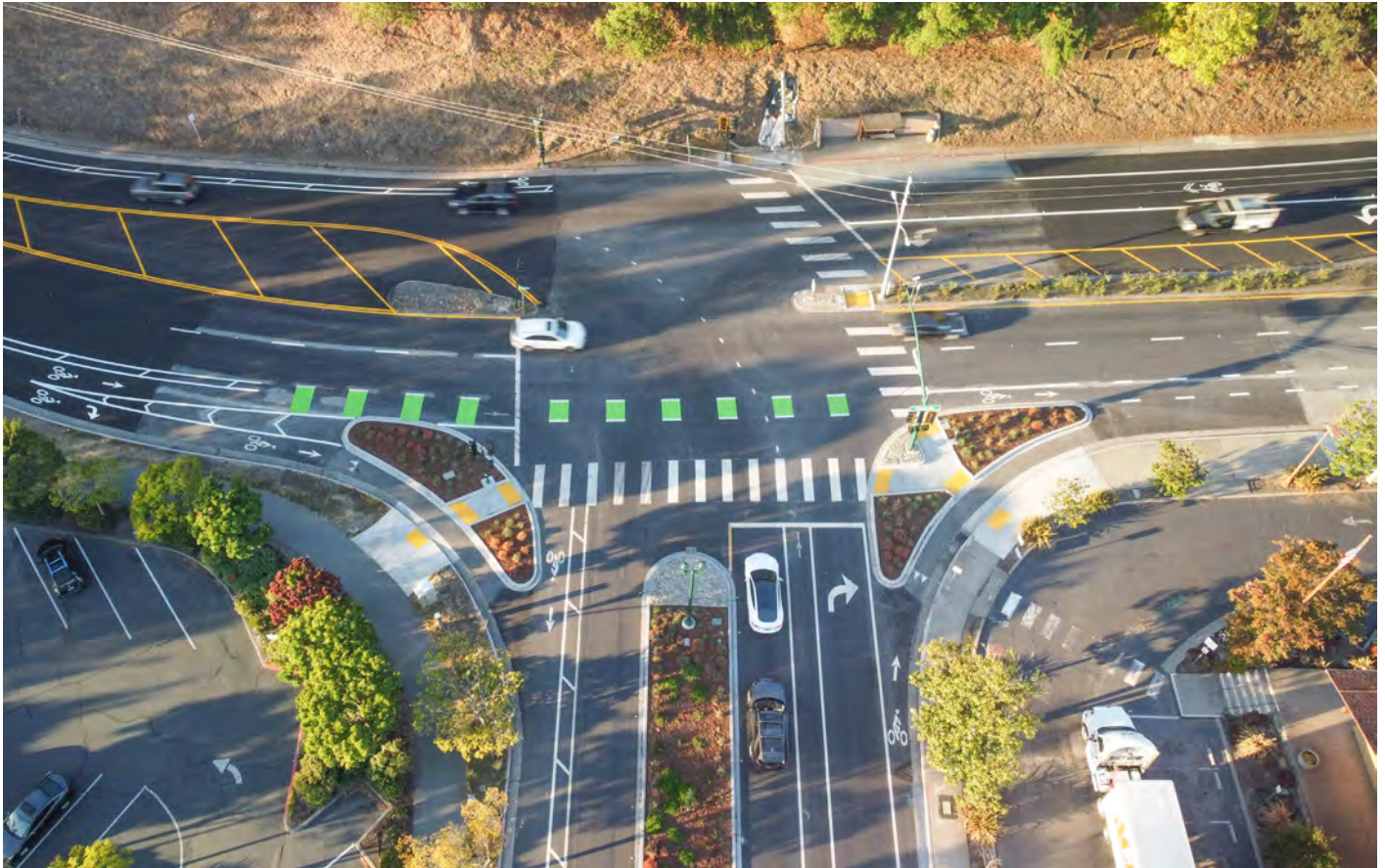
The Safe Routes Engineering program designs treatments to make it safer for students to walk and roll to school, such as this improvement to the Bon Air Road & Magnolia Avenue intersection in Larkspur.
