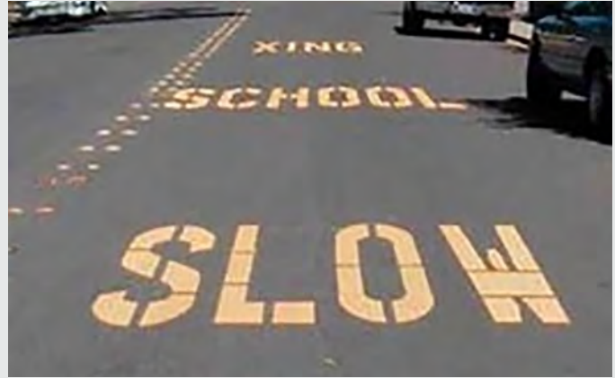
School area pavement markings also warn drivers that they are about to enter a school zone or encounter a school crossing.
