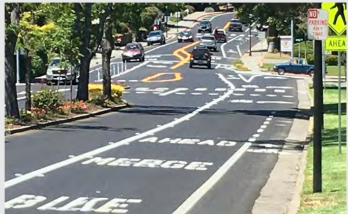
Bicycle lanes designate an exclusive space for cyclists through the use of pavement markings and signage. Bike lanes visually remind drivers of cyclists' right to the street.
