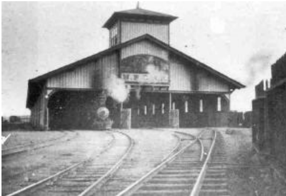
North Pacific Coast four truck train shed was erected on the pier at Sausalito in 1894. 324 feet long and 80 feet wide, big enough to allow passengers to transfer from trains to ferries under cover.
