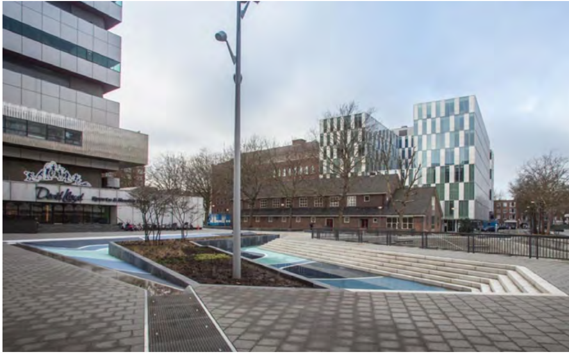
Figure 6: Submerged features in the public square can act as stormwater retention basins during flood events.
