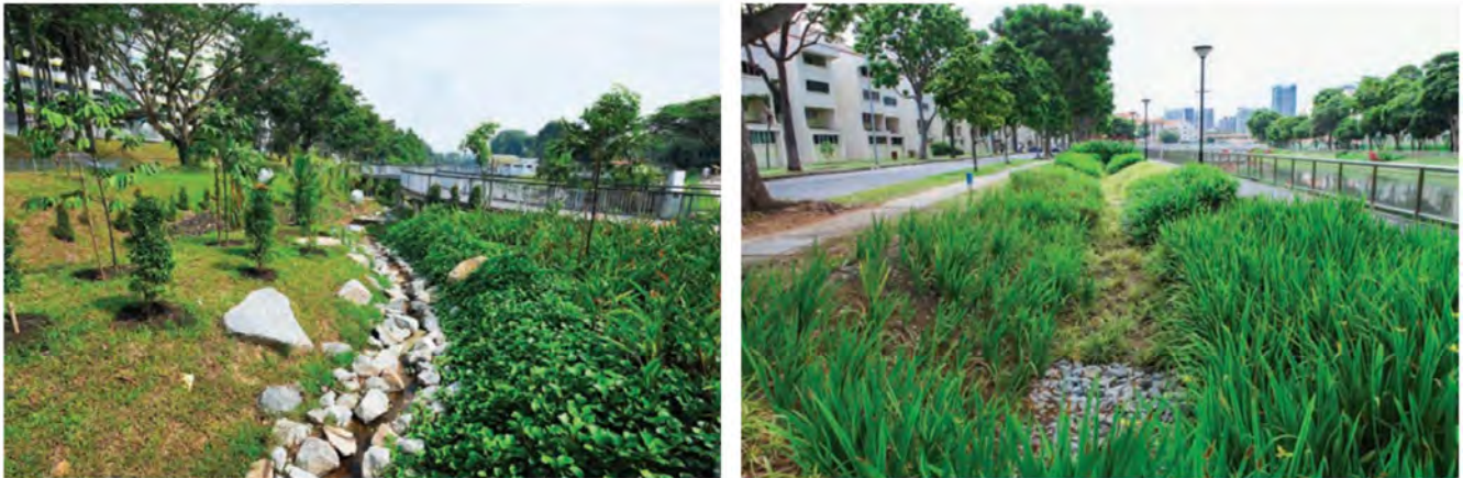
Figure 7: Natural drainage basins in Sg Ulu Pandan (left) and Kallang River at Potong Pasir (right) (ABC Waters).
