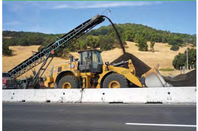
Construction is making great progress on the final section of HOV Lanes!
