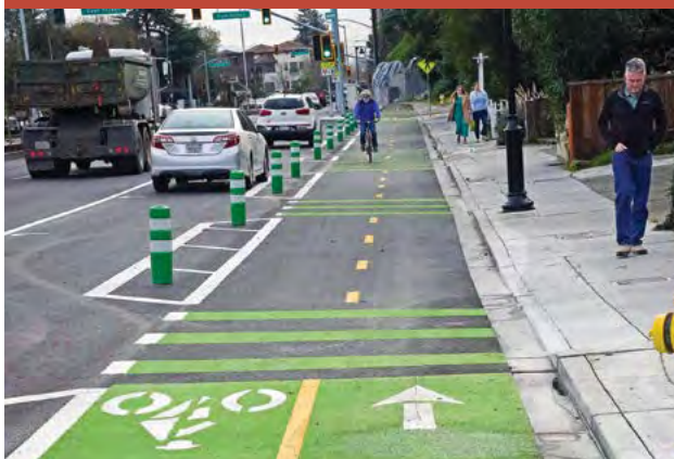
Third Street and East Blithedale Major Roads Projects complete!
