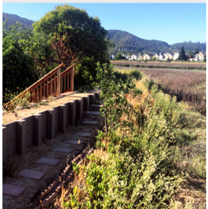
Marin County timber-reinforced levee system, August 2021. Photo by Marin County Public Works.
