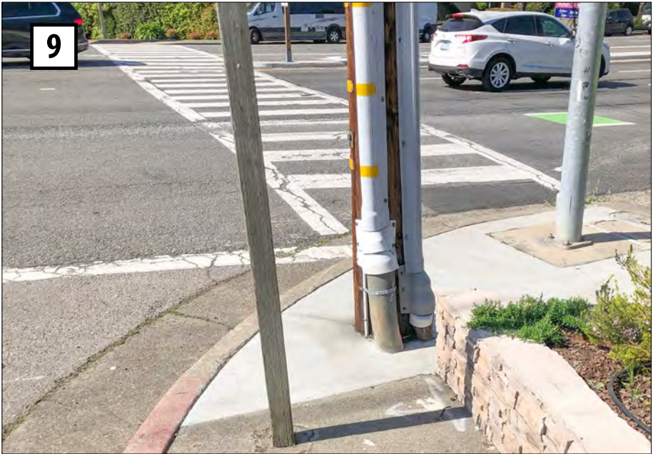
Uncontrolled crosswalk across Tiburon Boulevard at North Knoll Road; note lack of an ADA-compliant curb ramp.
