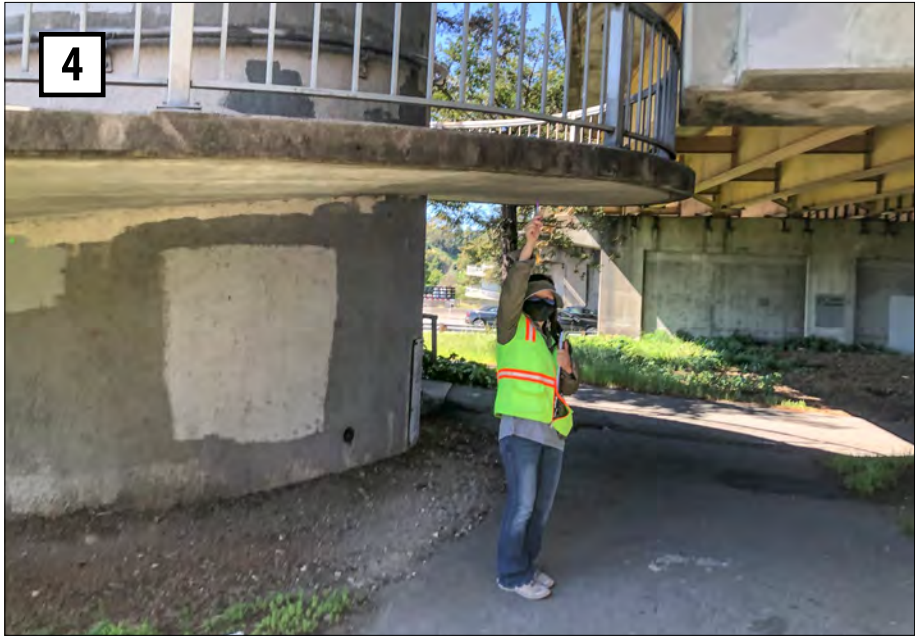
Spiral pedestrian ramp on the east side of Highway 101 connecting to the south side of Tamalpais Drive overcrossing; ramp grade exceeds ADA standards.
