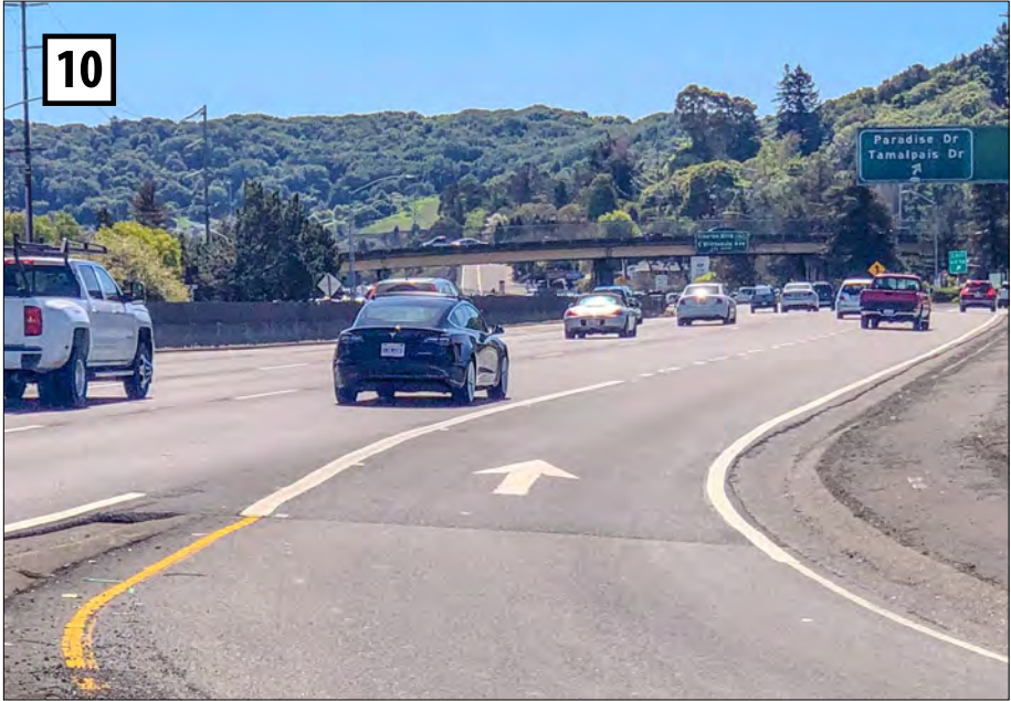
Weaving segment and auxiliary lane along southbound Highway 101 between the on-ramp from Madera Boulevard and the off-ramp to Tamalpais Drive.
