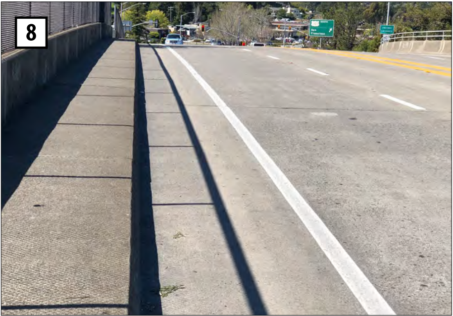
Sidewalk, shoulder, and eastbound vehicular travel lanes on Tamalpais Drive overcrossing; note the structure's vertical crest curve.
