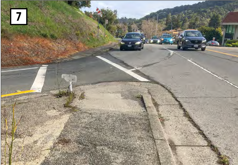
Looking east on the north side of North San Pedro Road at entry to Highway 101 northbound on-ramp; walkway and sidewalk are not in compliance with ADA standards.
