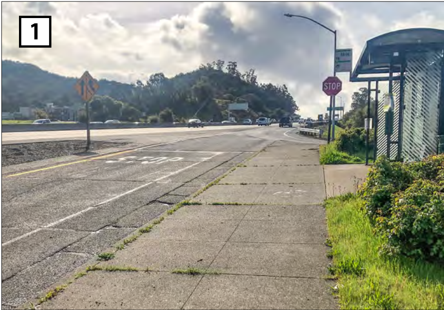
Bus stop along Highway 101 northbound; platform and sidewalk grade exceed ADA standards.
