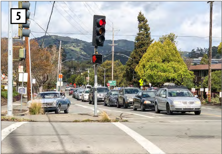
Southbound traffic queued along Merrydale Avenue's approach to North San Pedro Road; note pedestrian crosswalk and non-ADA-compliant curb ramp.
