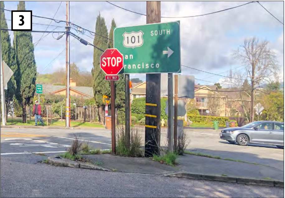
"Pork chop" island at southeast corner of Merrydale Avenue and Highway 101 southbound ramps terminal, walkway leads into utility pole and sign posts.
