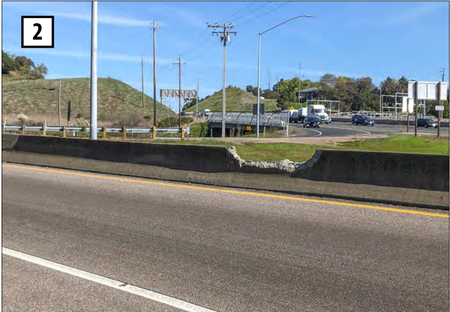
Broken divider separating the southbound off- and on-ramps with sidewalk serving the southbound Highway 101 bus stop.
