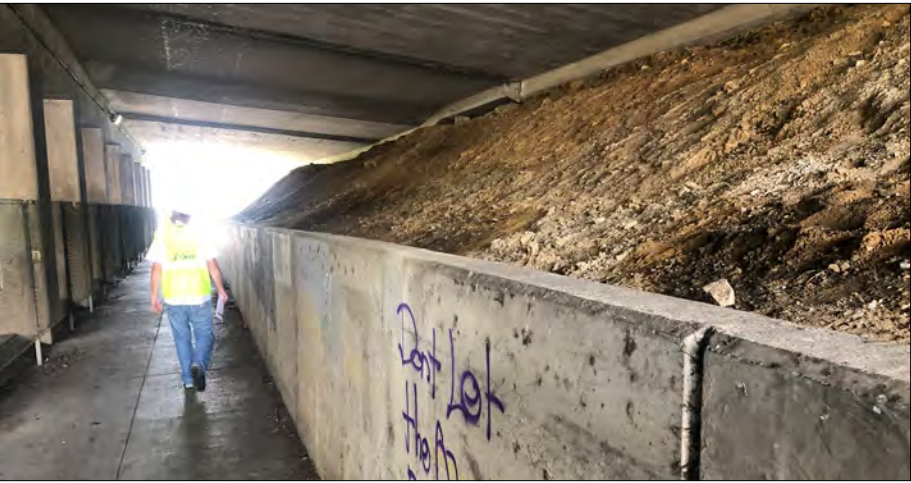
Retaining wall along the sidewalk under the Highway 101 overcrossing; provision of a new wall to the south could enable a wider active transportation facility.
