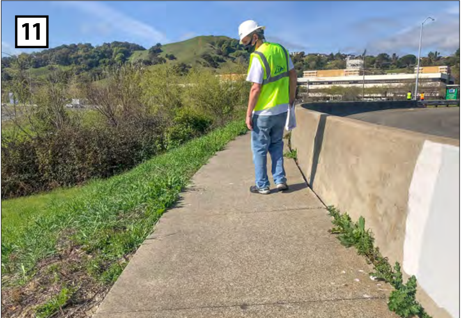
Sidewalk serving the Highway 101 northbound bus stop; the sidewalk is peripheral to the northbound loop on-ramp and its cross-slope exceeds ADA standards.
