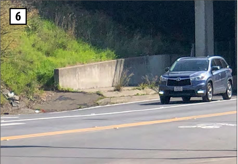
Westbound bicyclists crossing under Highway 101 use a nonstandard separated bikeway with a ramp merging with Lucas Valley Road.
