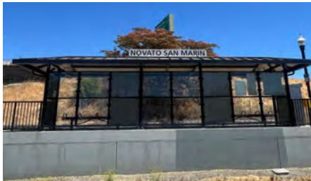
San Marin SMART Station
