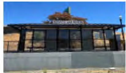
San Marin SMART Station
