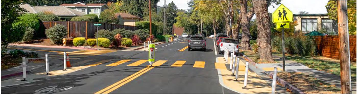
Safe Routes engineering improvements include quickbuild options such as these upgrades on Magnolia Avenue in Larkspur..
