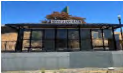
San Marin SMART Station
