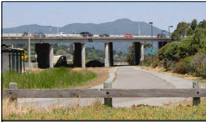
The former rail Right of Way (RoW) offers a non street-running alternative to Bridgeway, but requires shared use of the RoW with a Class I bike trail. The rail alignment passes under Hwy 101, avoiding a challenging roadway crossing of Hwy 101 and several signalized intersections on the street running alignment on Shoreline/Tam Junction. The support columns for Hwy 101 have crash protection installed for previous rail operations.
