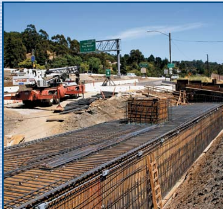
Puerto Suello Hill Multi-use Path Tunnel Under Construction.
