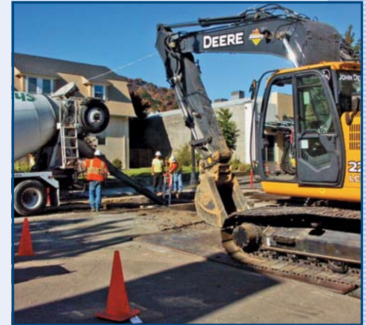
San Rafael 4th Street Project Construction Site.
